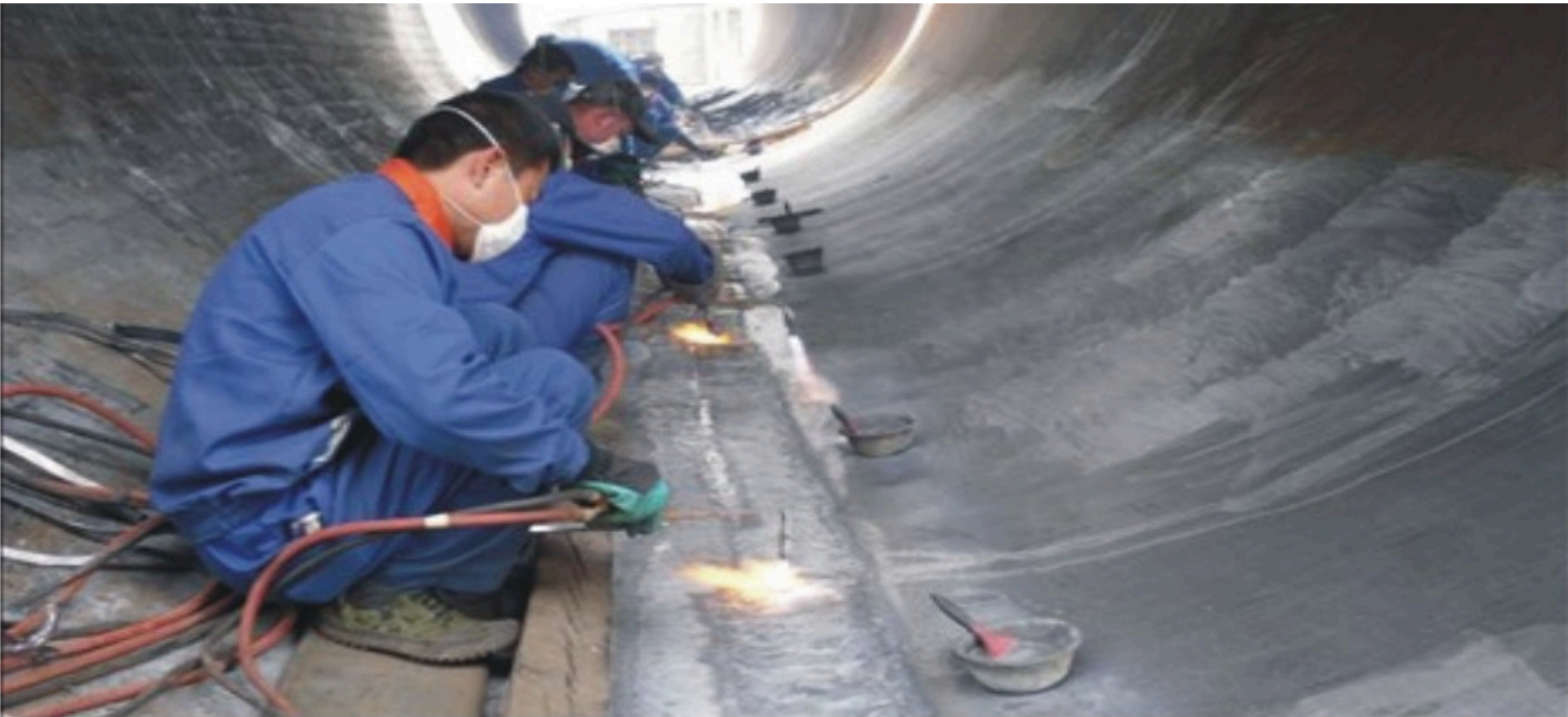
Construction site of 100Kt/a electric zinc oxygen pressure leaching high-pressure reactor
