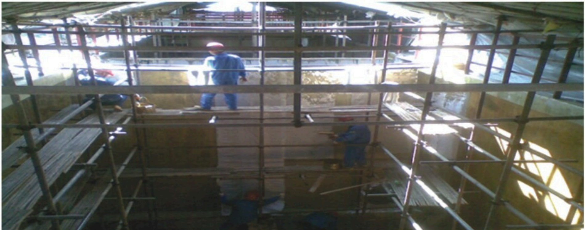
55kt/a neutralization and oxidation tank FRP anti-corrosion stage
