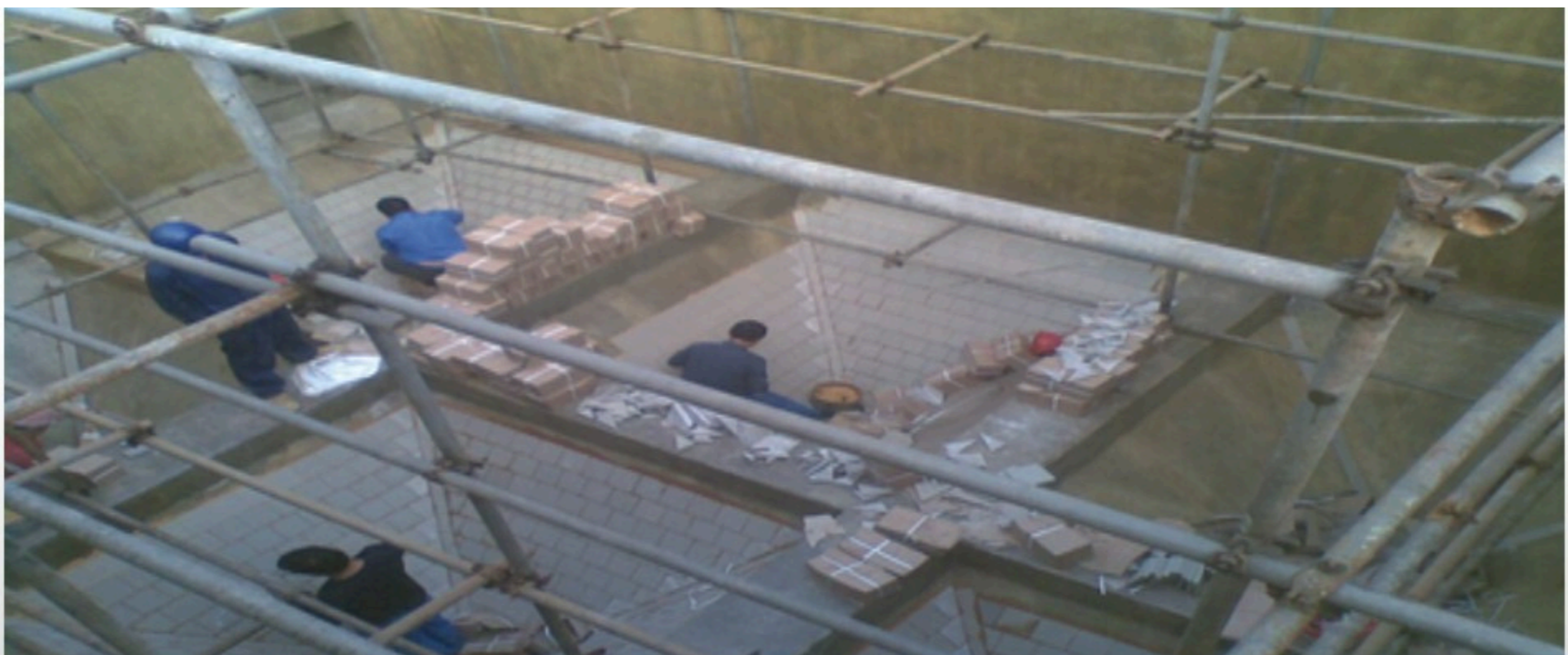
55kt/a neutralization oxidation tank lining brick anti-corrosion stage
